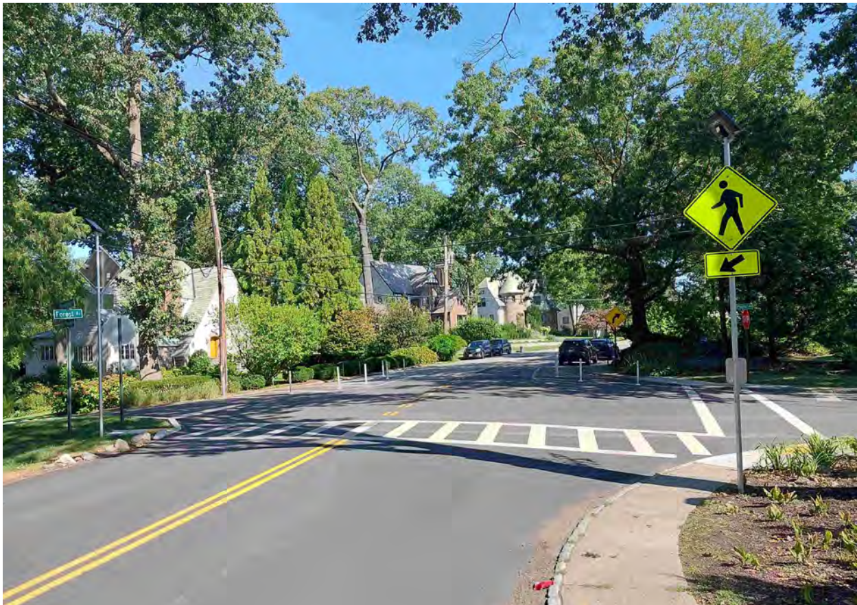
New Rochelle Traffic Calming Program Improvements (Source: New Rochelle)
