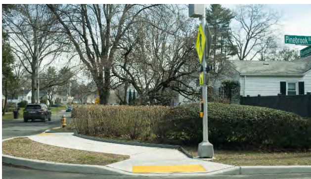
ADA-compliant Pedestrian Signal and Curb Ramp on Pinebrook Boulevard
