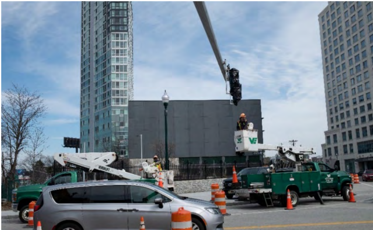
New Traffic Signal Installation on North Avenue
