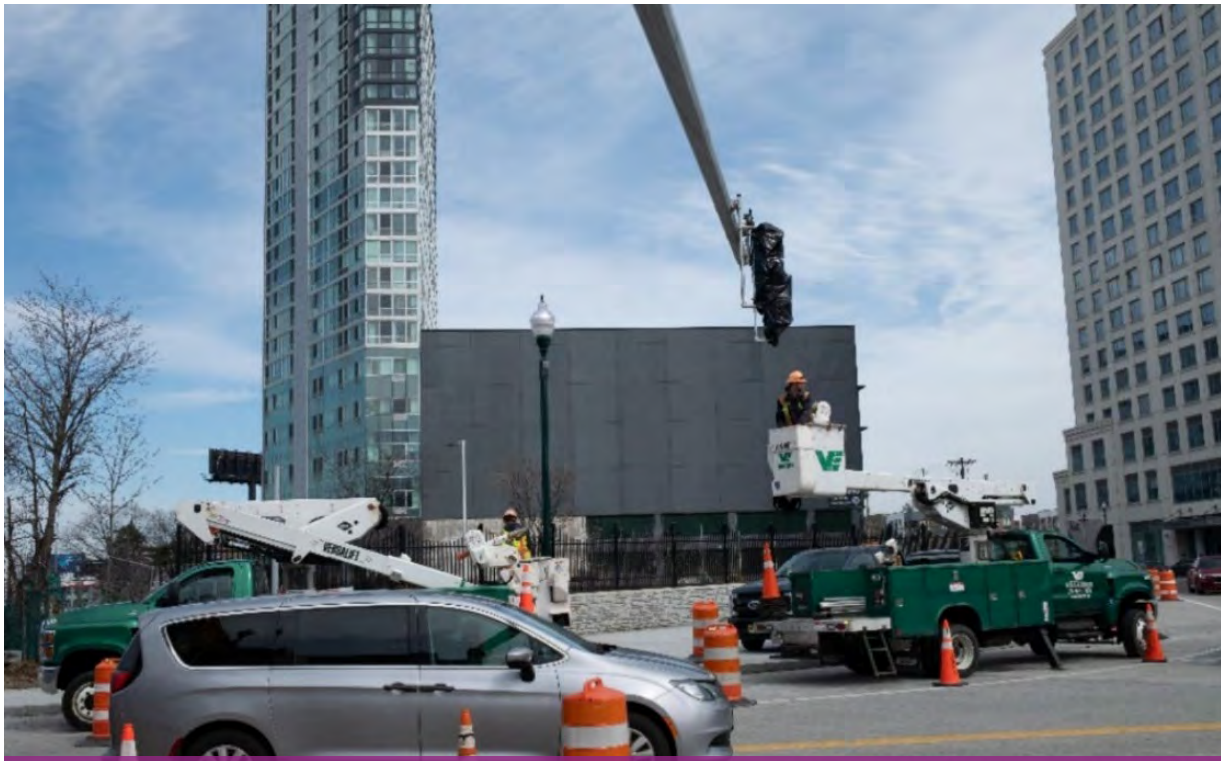
New Traffic Signal Installation on North Avenue
