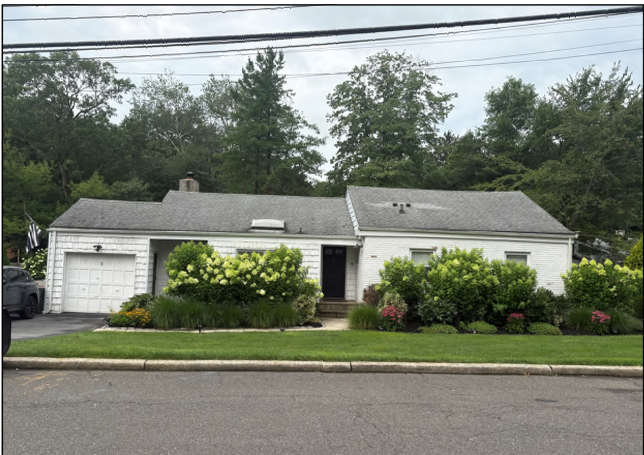
8 HIGHRIDGE ROAD FRONT ELEVATION
