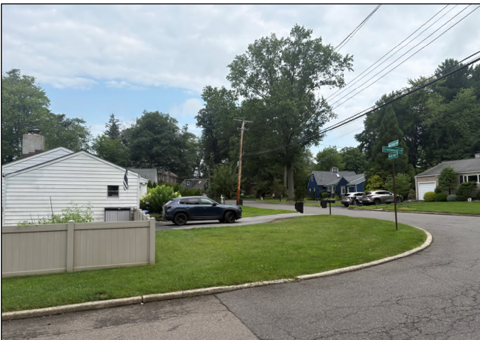
8 HIGHRIDGE ROAD SIDE ELEVATION
